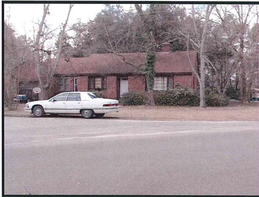
West view from site (Site 2)
